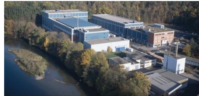
ZWILAG Intermediate Storage Facility, Switzerland
