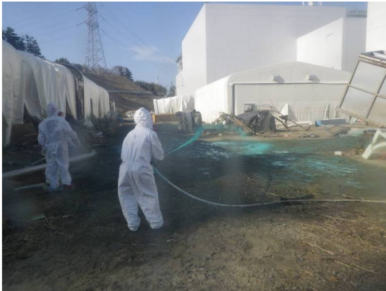
Spraying dust inhibitor agents
