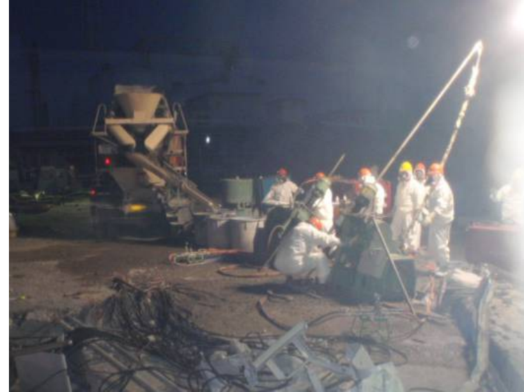
Coagulant injection to stop outflow
